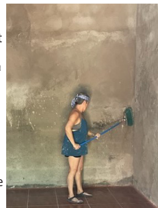
Marie prepping interior walls
